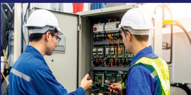
Electrical and mechanical installation
